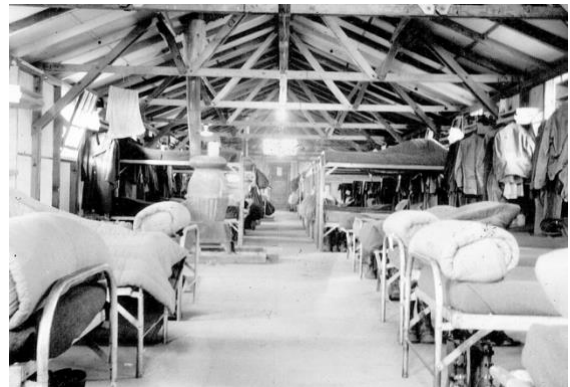
Wendover barracks during 384th training, 1943
