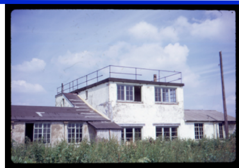
Grafton Underwood Control Tower 1973 Photo by Paul Knight, sent by Kevin Flecknor
